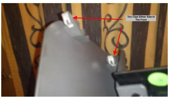
Push in the plastic lugs with small screwdrivers or plastic tools and hook something like coat hanger wire under the cutouts to draw the socket out from the surround (or a bit of string under the rim)
